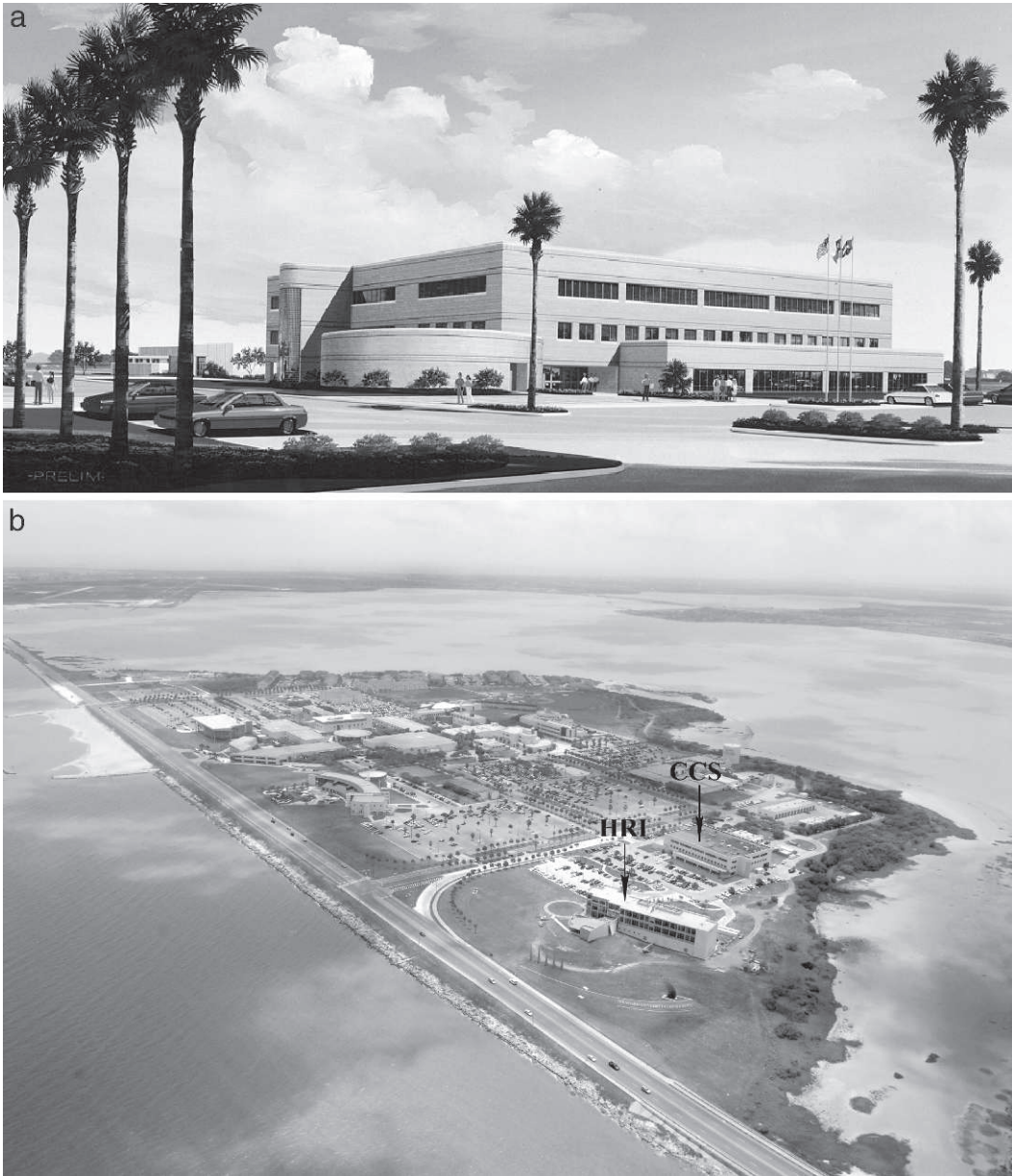
Fig. 3. Carlos F. Truan NRC on the TAMU-CC campus: (a) artist's rendering and (b) aerial view to the southeast of the Ward Island campus between Corpus Christi Bay (left) and Oso Bay (background) showing the NRC building that houses the CCS and the HRI for Gulf of Mexico Studies (Photos courtesy of TAMU-CC).
